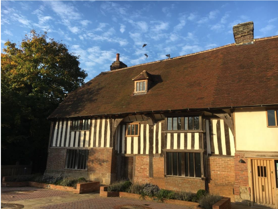
ABOVE: THE NEW LOOK BRIDGE COTTAGE
